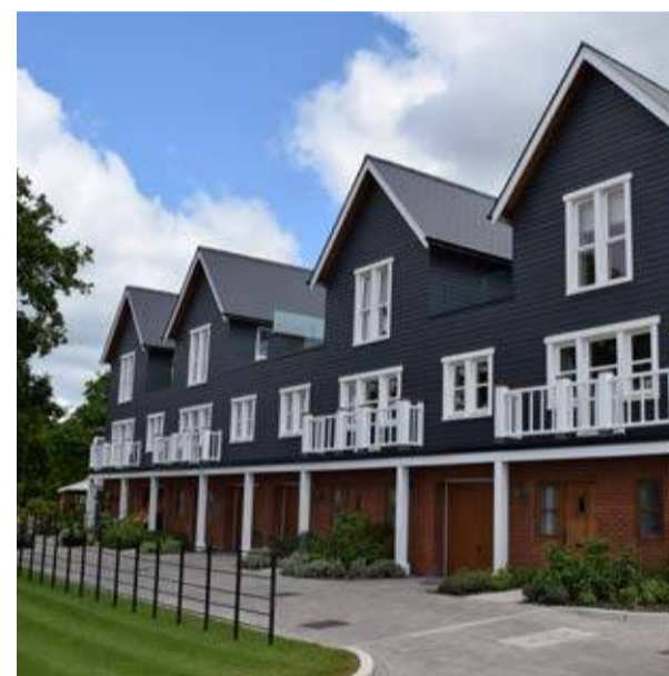
Continuous frontage and contemporary take on traditional terrace design elements.
