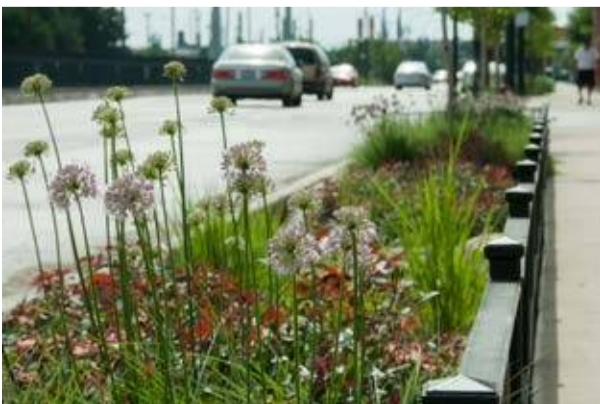
Rain gardens in the streetscape
