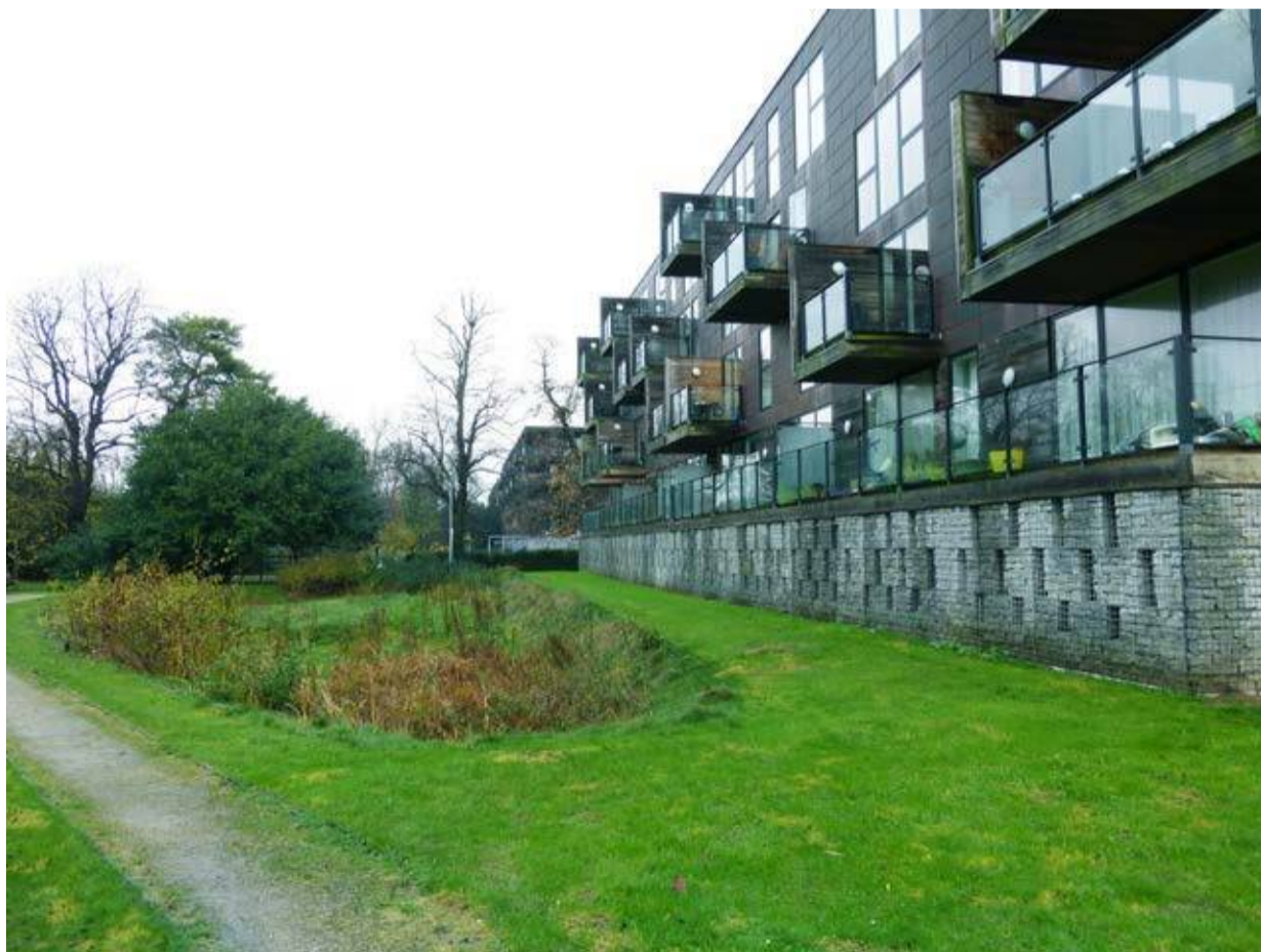
An example open space overlooked/enclosed by taller built elements (Accordia, Cambridge).
