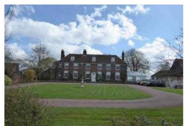
Principal south elevation fo the Dunton Hills farmhouse
